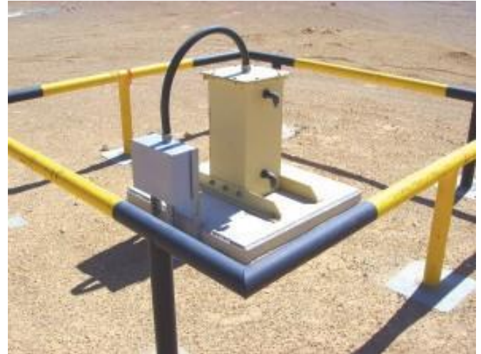
Anode Junction Box fixed with steel support mounted on concrete foundation at anode deep grounded structure
